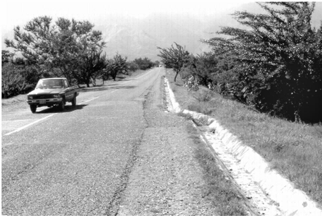
Fig. 28 - C.A. 10, toward Estanzuela: sinistral offset of the drainage crossed by the Cabañas fault, as NOAM- CARIB Plate border.
